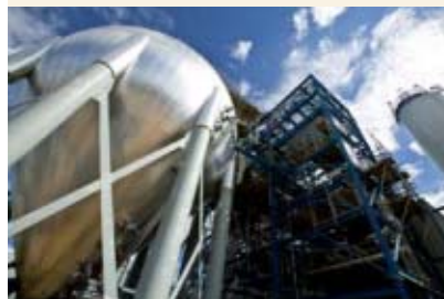
Using saline water for steam.
