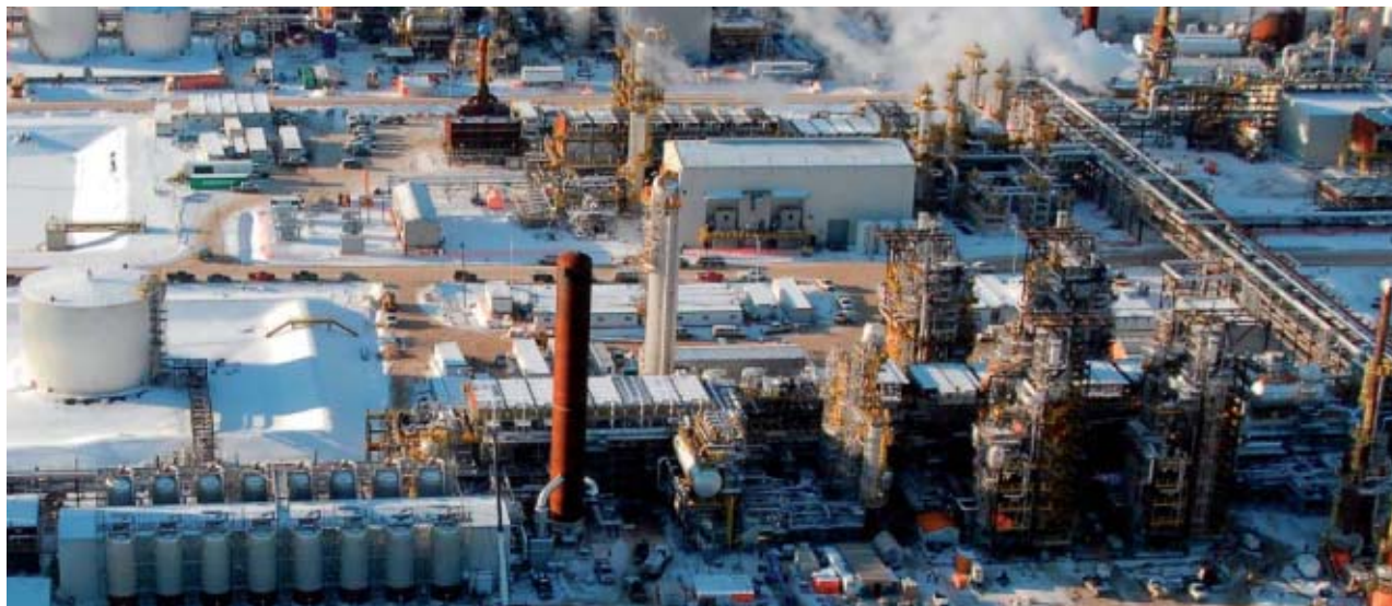
Gasifier and Hydrocracker, Long Lake Project.
