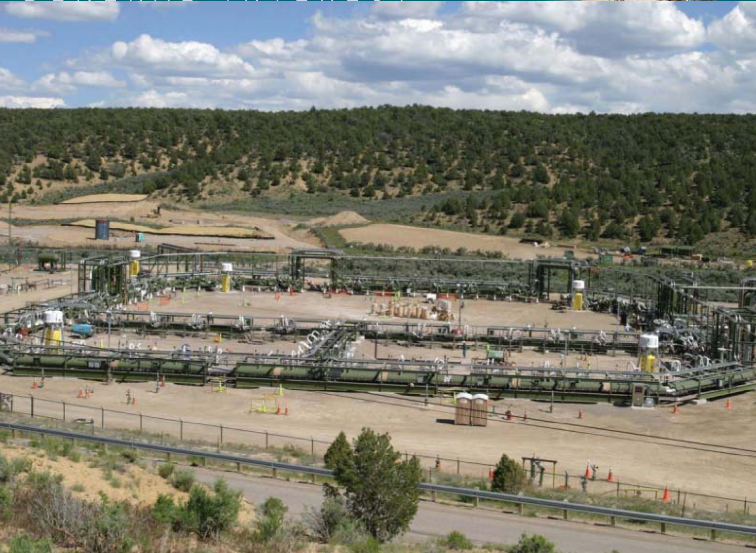
Shell's Freeze Wall test site at its Mahogany Research Project in Rio Blanco, County, Colo., involves a vertical ice wall and contained oil shale reservoir to prevent ground water contamination. Freeze began in early 2007. Photo from Shell Exploration & Production Co. Unconventional Oil.
