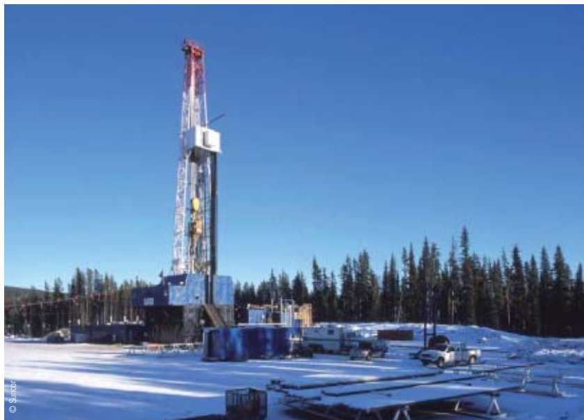
Natural Gas rig.
